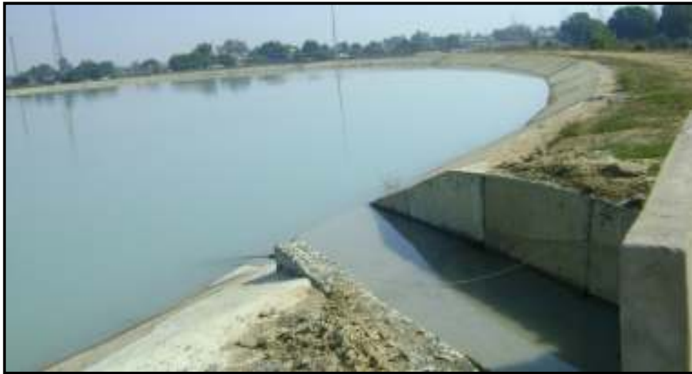
Ash Dyke Pond
