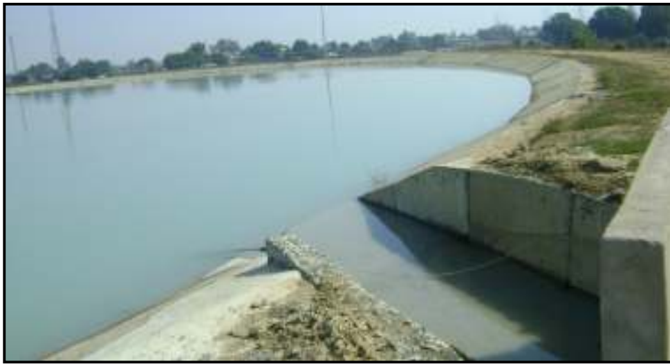
Ash Dyke Pond
