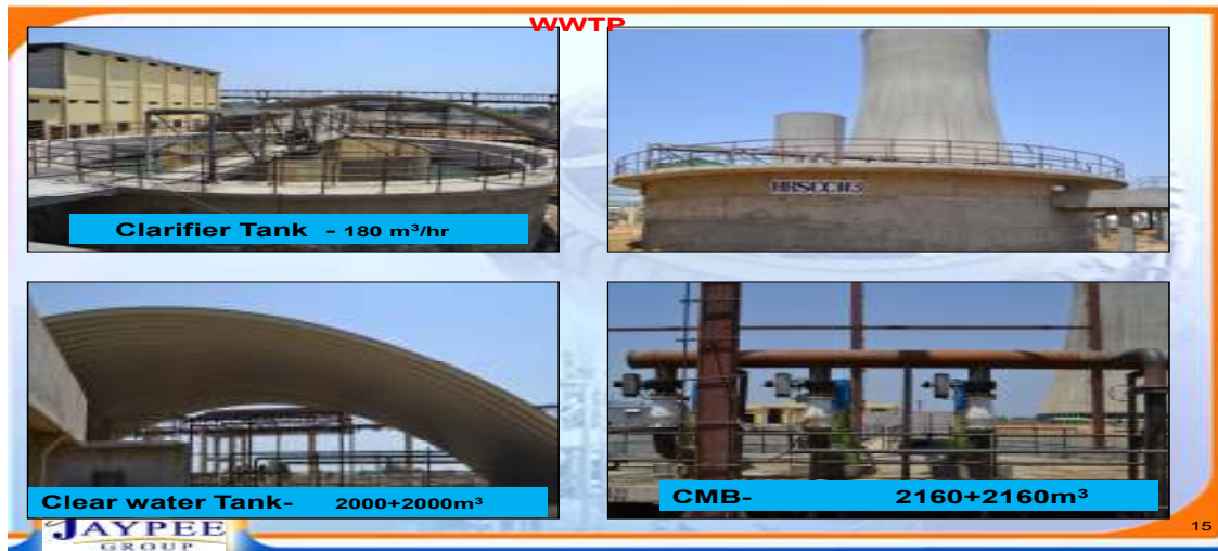
Photograph of WWTP
