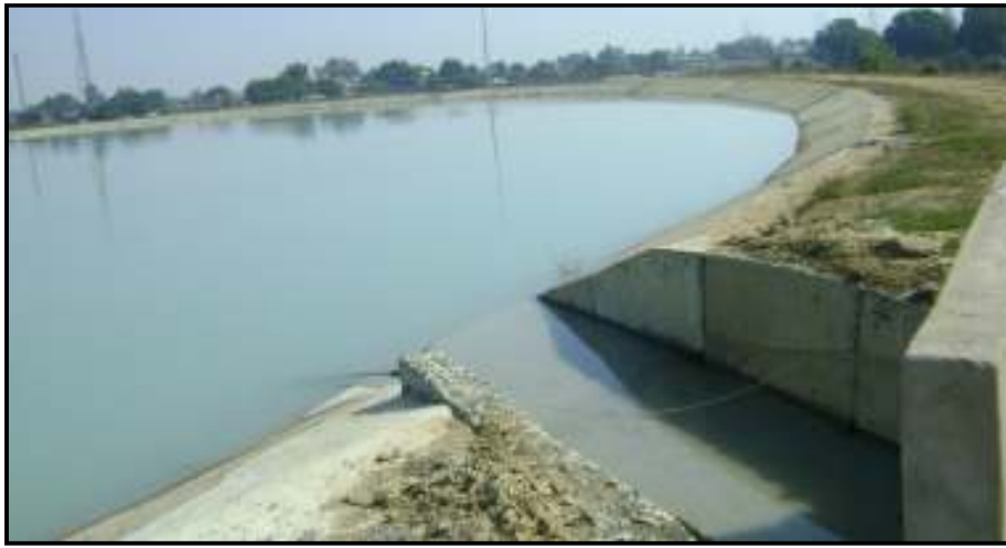
Ash Dyke Pond
