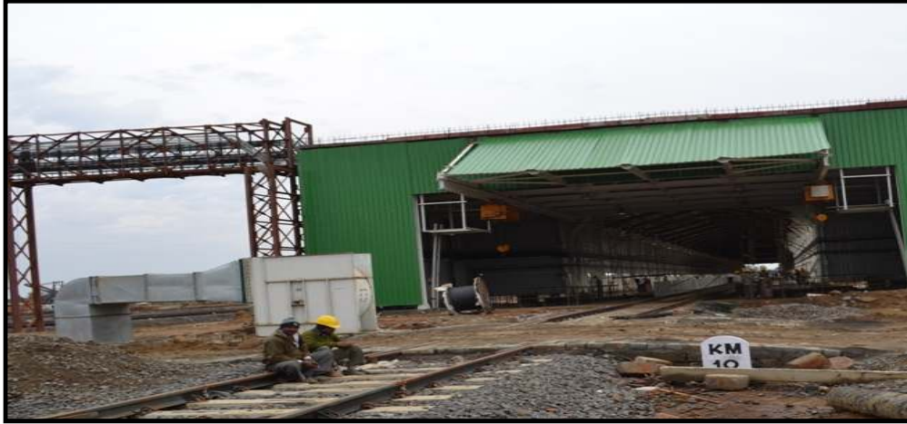
Coal wagon unloading system
